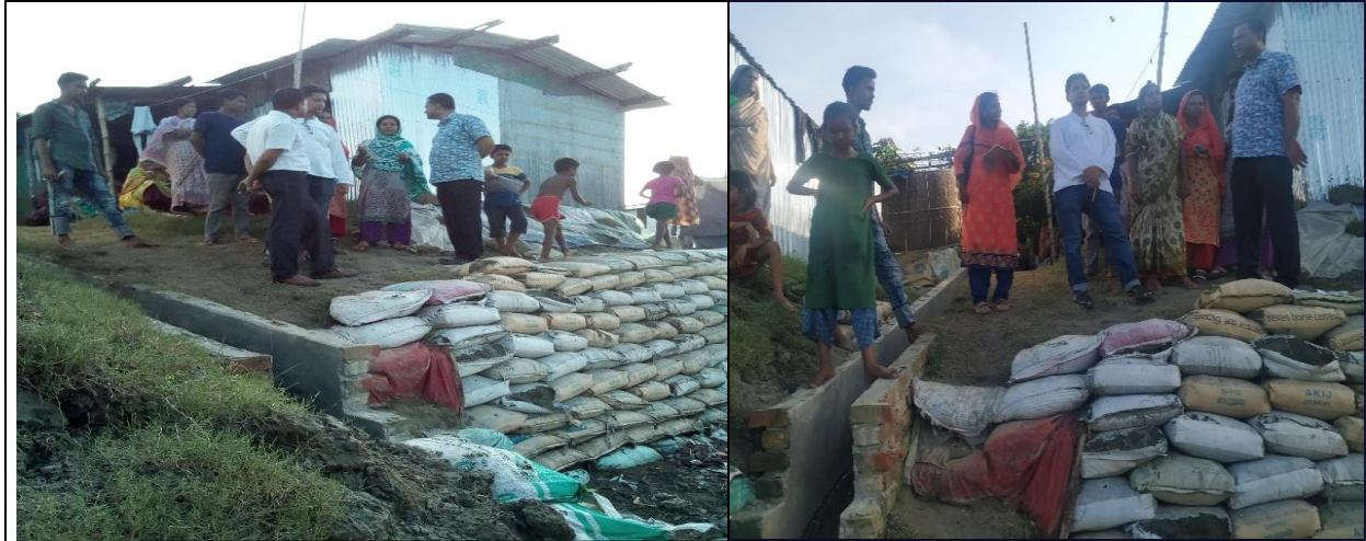
Construction of Embankment
